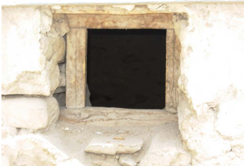
1.5 A poorly constructed cattle shed window. Openings are larger than 4"x 4", possibly large enough to allow a snow leopard inside.
