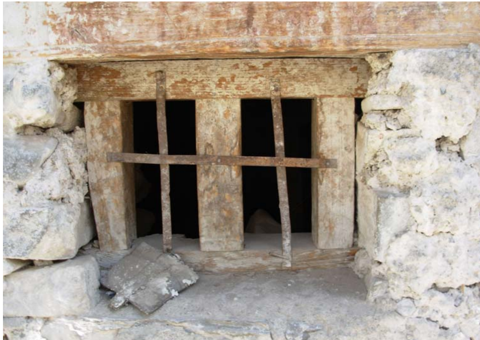
1.6 A well-constructed cattle shed window. Openings are smaller than 4"x 4" and protected by metal strips.
