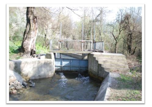
Plate 52. Water supply department control gate and canal
